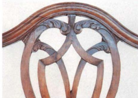
*Weak cross grain on the crest rail of this old chair is prone to breakage, especially when it's mortised to accept the tenon of the chair back.*
