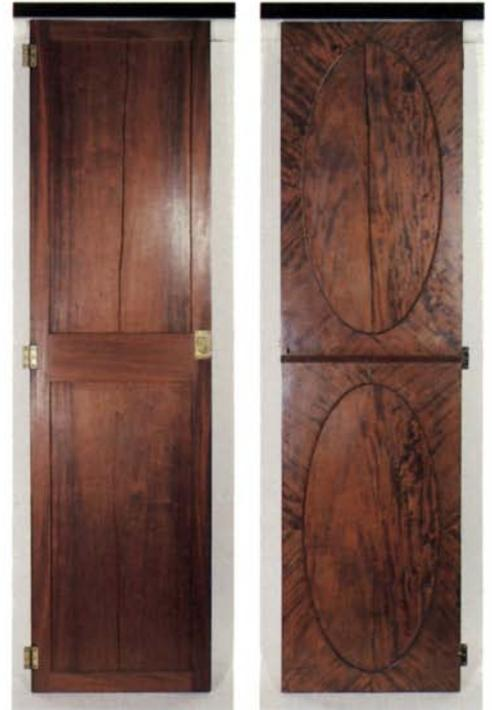
*Large splits shouldn't occur in floating-panel doors. But the back side of this door reveals that either glue used to attach the decorative veneer panels or shellac applied to the door locked the panels in place. Normal wood movement then split the panel.*
